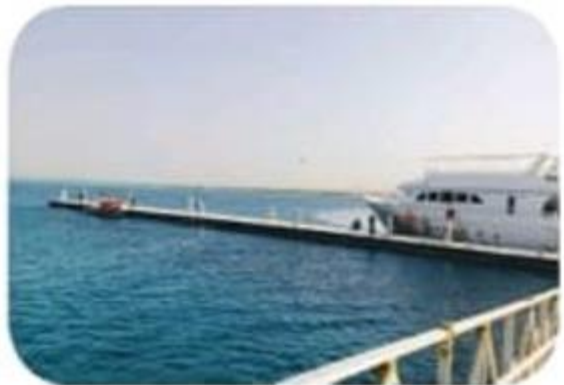
TAWILA ISLAND DOCK
